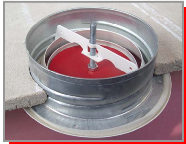
Fire Air Valve installed before a fire
